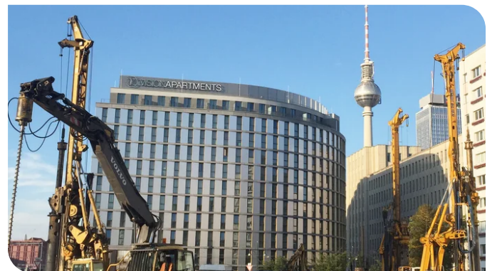
Large drilling rigs during the construction of bored piles. Image: PORR AG
