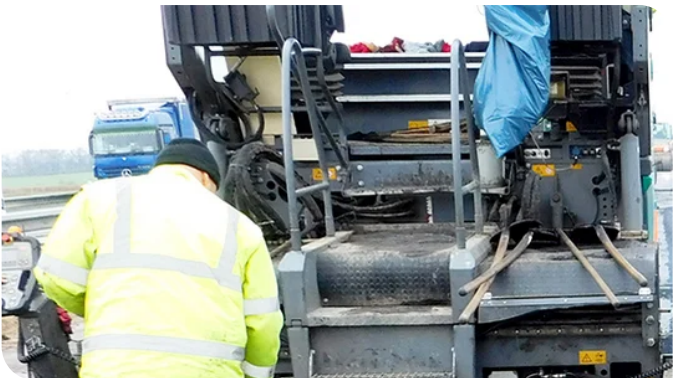
RB 500 resonance crusher - construction machine for demolishing the concrete substructure. Image: PORR AG
