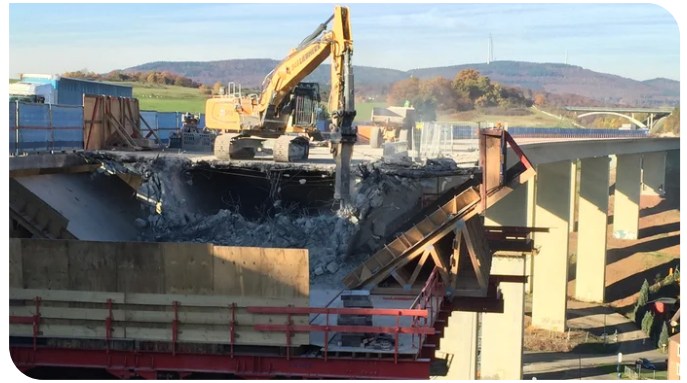
The demolition work was carried out using an excavator. Image: PORR AG
