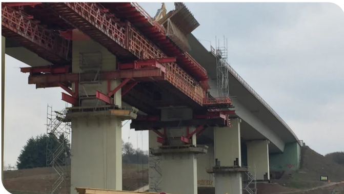
The new bridge piers, axis 50 and 60, are between 15.5 m and 35 m high and were concreted in individual sections of 5 m each. Image: PORR AG
