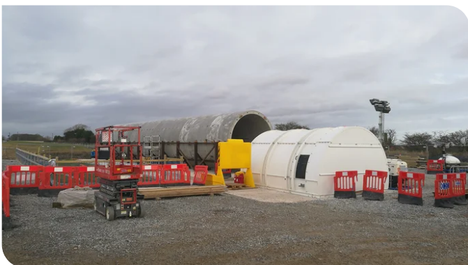
The tunnel mock-up for training purposes. Image: PORR AG
