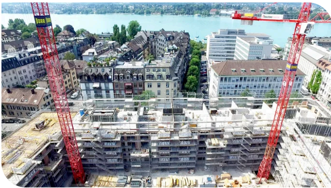
PORR employed a mixture of traditional load-bearing outer wall construction techniques for the upper floors. Image: PORR AG
